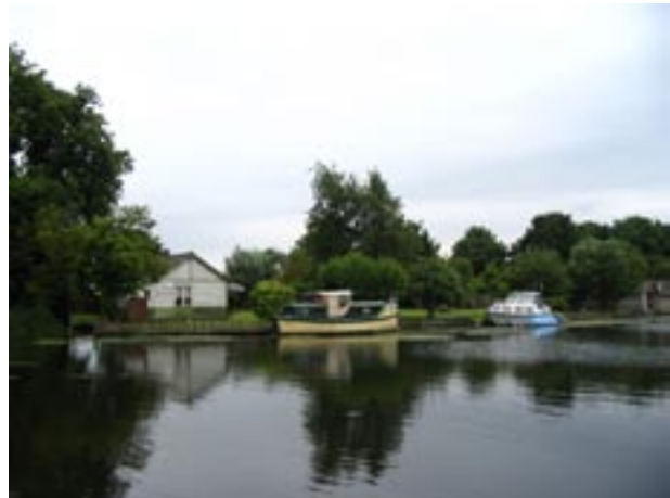
View to timber-boarded boathouses
