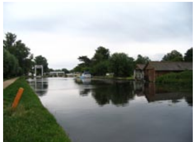
View downstream towards the lock
